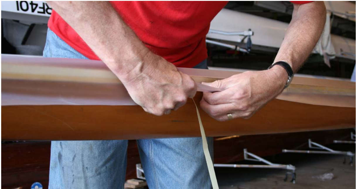
Figure 12: Making the second joint. The boatman applies crosswise tension, and a little lengthwise to match the tension in the middle, and then presses the material firmly onto the tape. This is our earlier one-man technique; later we had a second person pressing the material onto the tape while this first one did the stretching.
