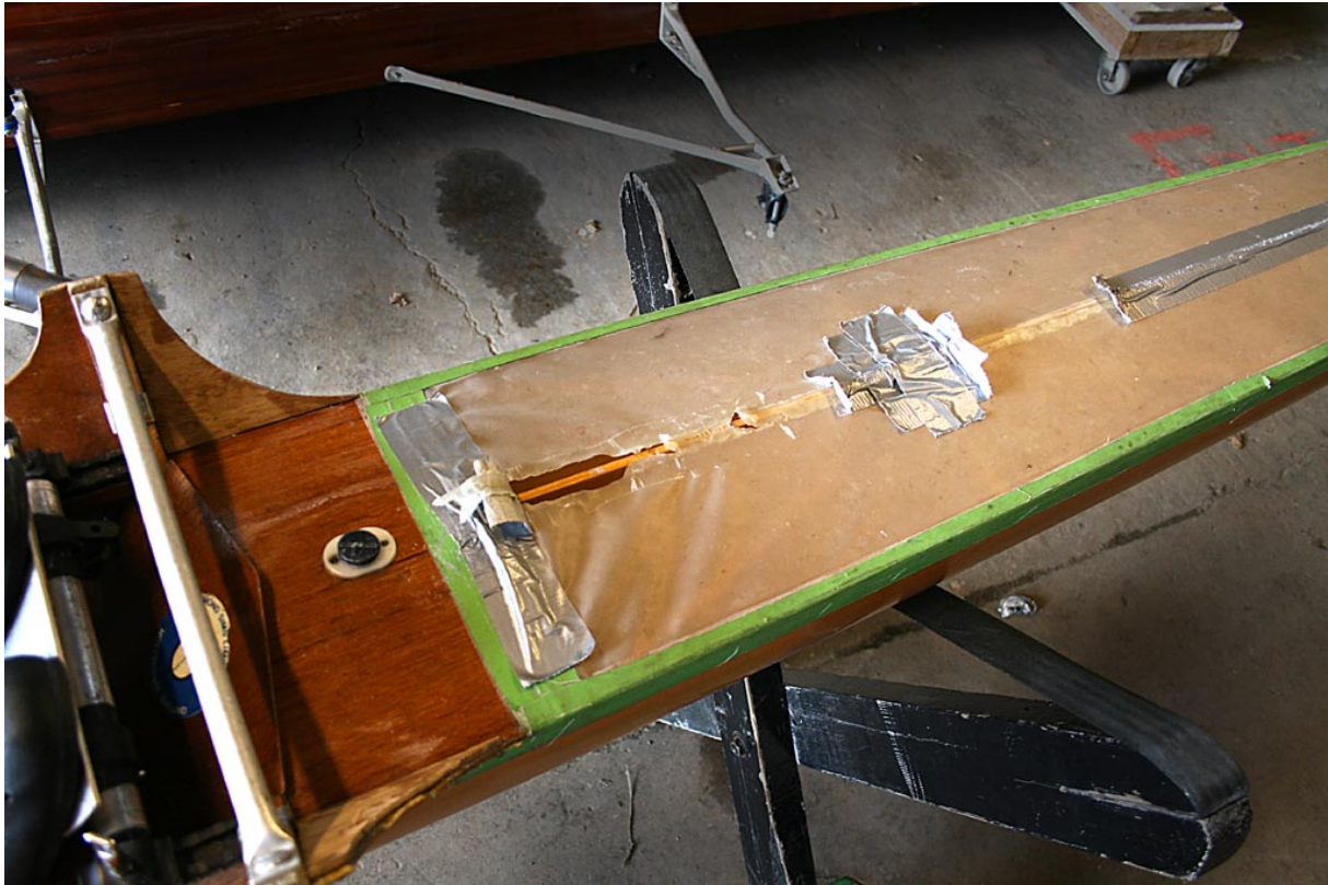
Figure 1: Damage to the old decking
